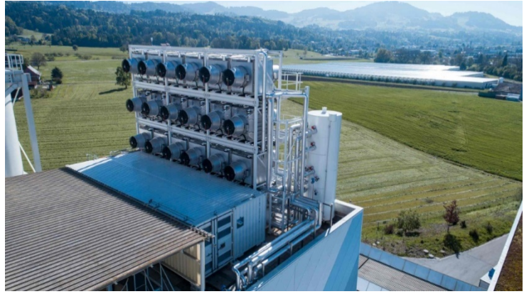
This image shows the fans of the Swiss Co2 Capture System -From Climate Central
